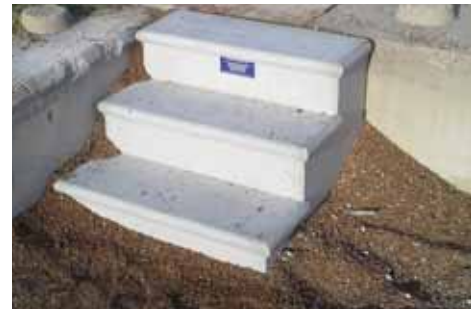
New steps installed at the swim beach area.
