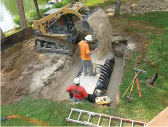
Installation of a residential STEP tank requires a minimum of six inches of compacted gravel on all sides.
