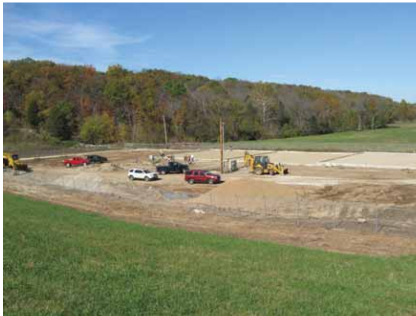
View of the treatment plant from the top of the dam.
