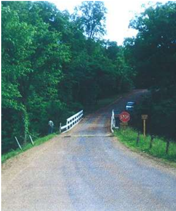
The one-lane bridge crossing the inlet creek (looking southwest)
