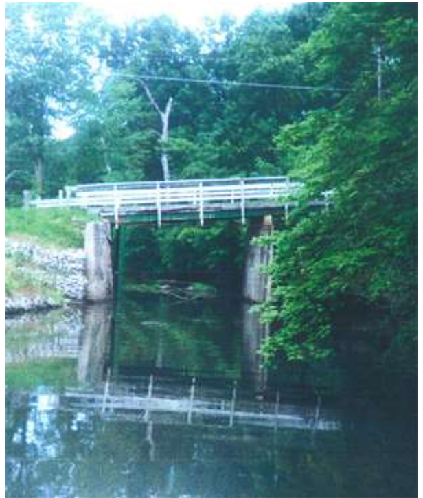
Bridge viewed from the lake side
