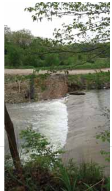
New spillway weir after repair.
