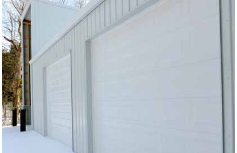
New maintenance building with two garage doors and large open bin for salt storage.
