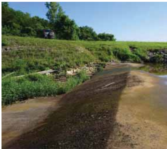
Weir looking towards dam, 6/2/2017
