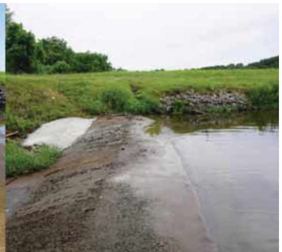
Weir, after repair, looking towards dam, 6/14/2017
