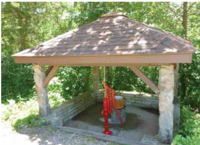
Pump house recently remodeled by the Lakeside Gardeners.
