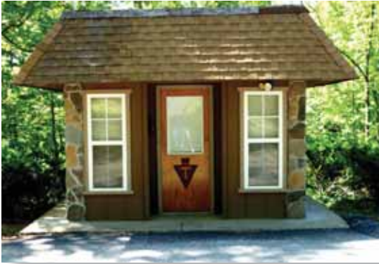
The Guard Shack newly remodeled by the Lakeside Gardeners.
