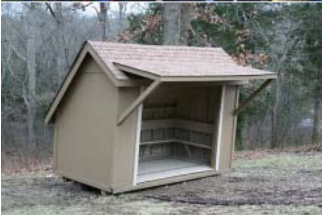
The bus shelter renovation.
