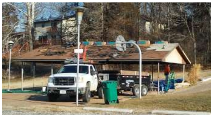
Working on the pavilion
