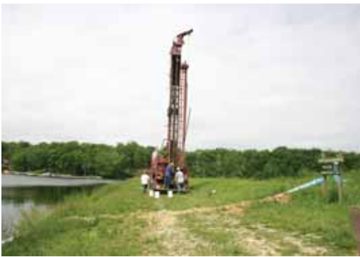
Drilling exploratory holes.
